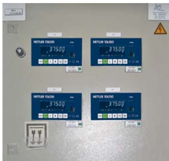
Raw material batching with PTPN process terminals
